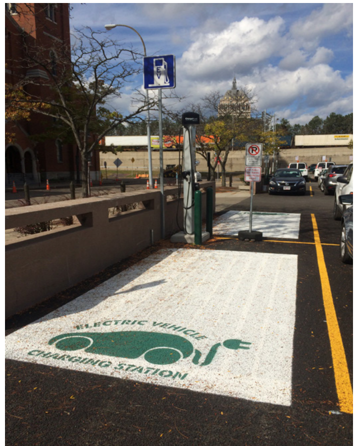
Electric Car Charging Station
